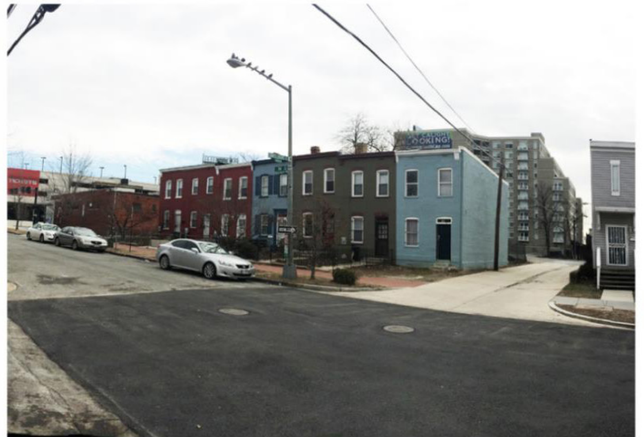
ROW HOUSES ON N STREET
